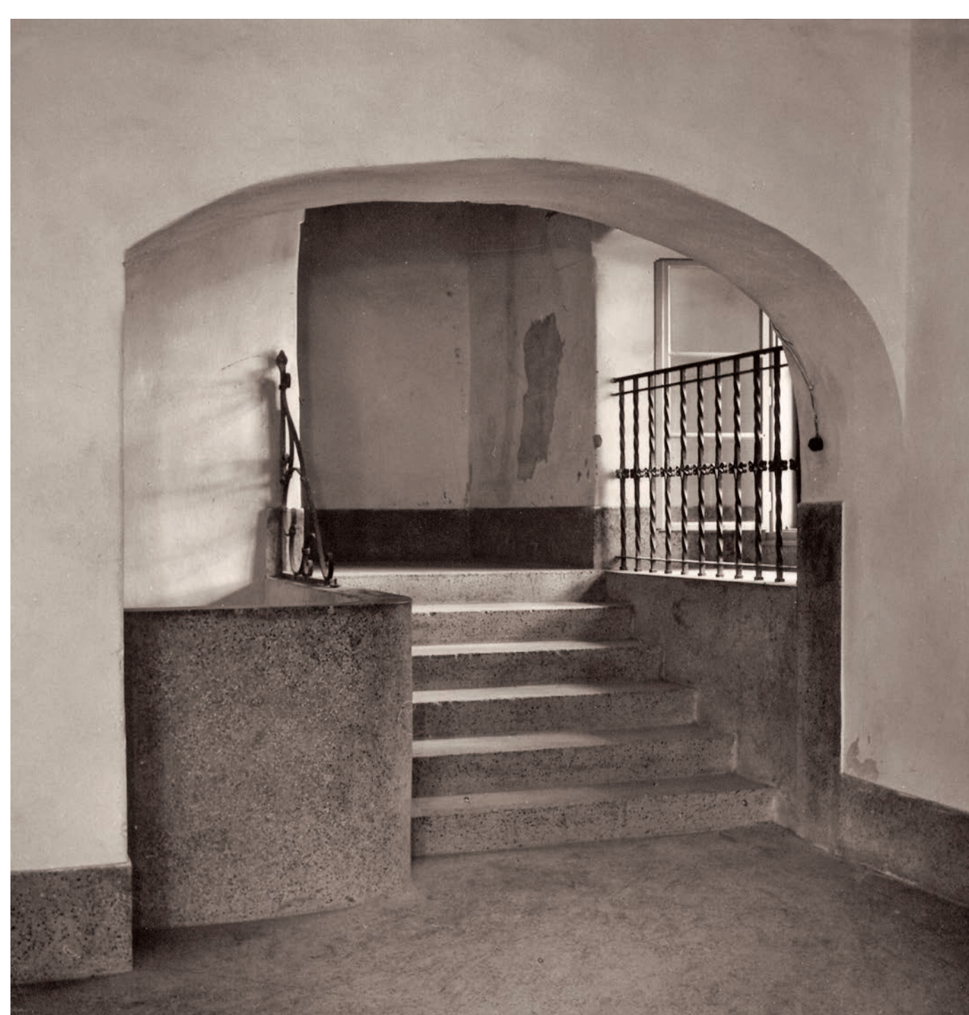
Betonsko stubište, 1954. / Concrete stairway, 1954
