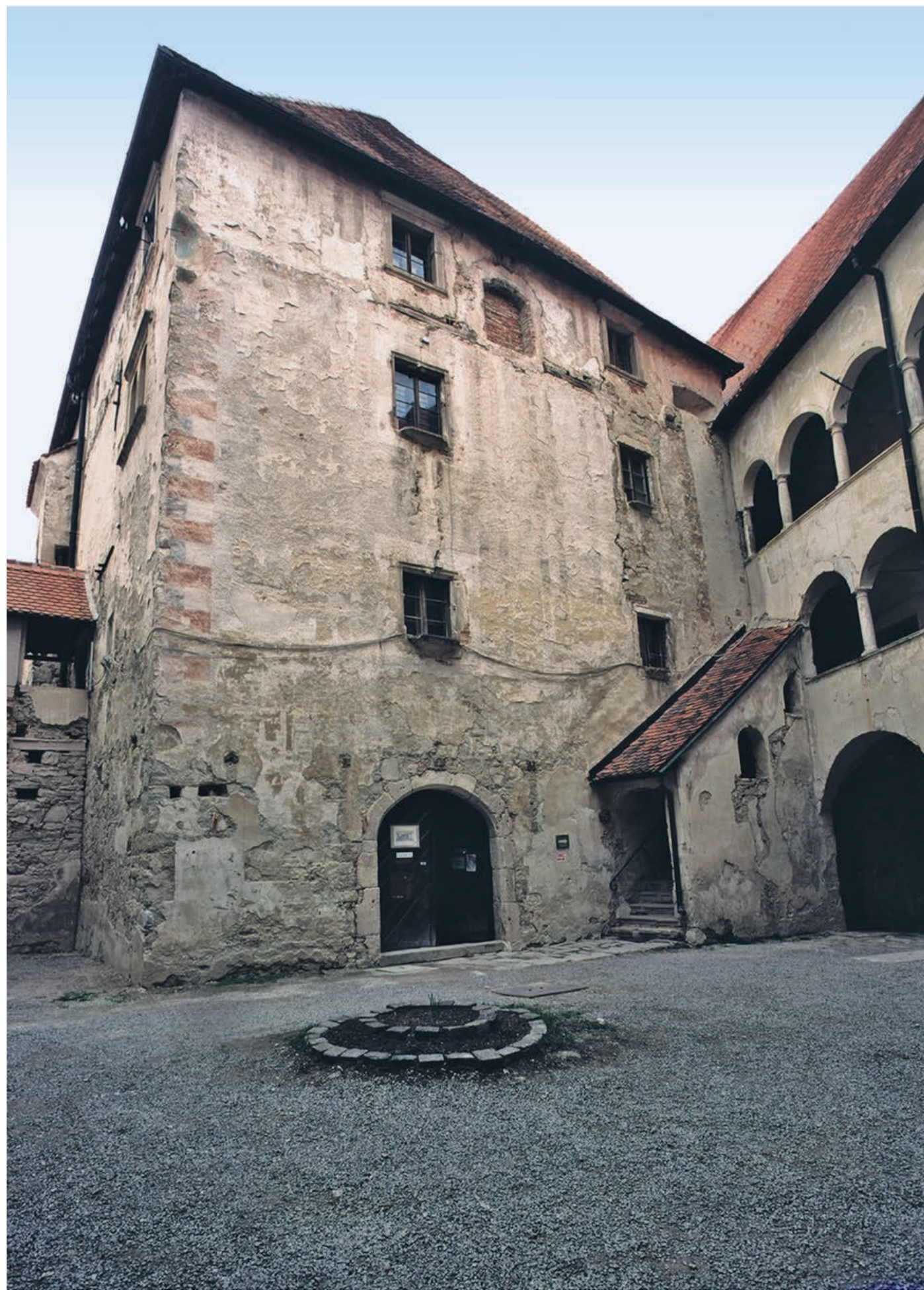
Veliki Tabor prije radova obnove Veliki Tabor before the reconstruction works
